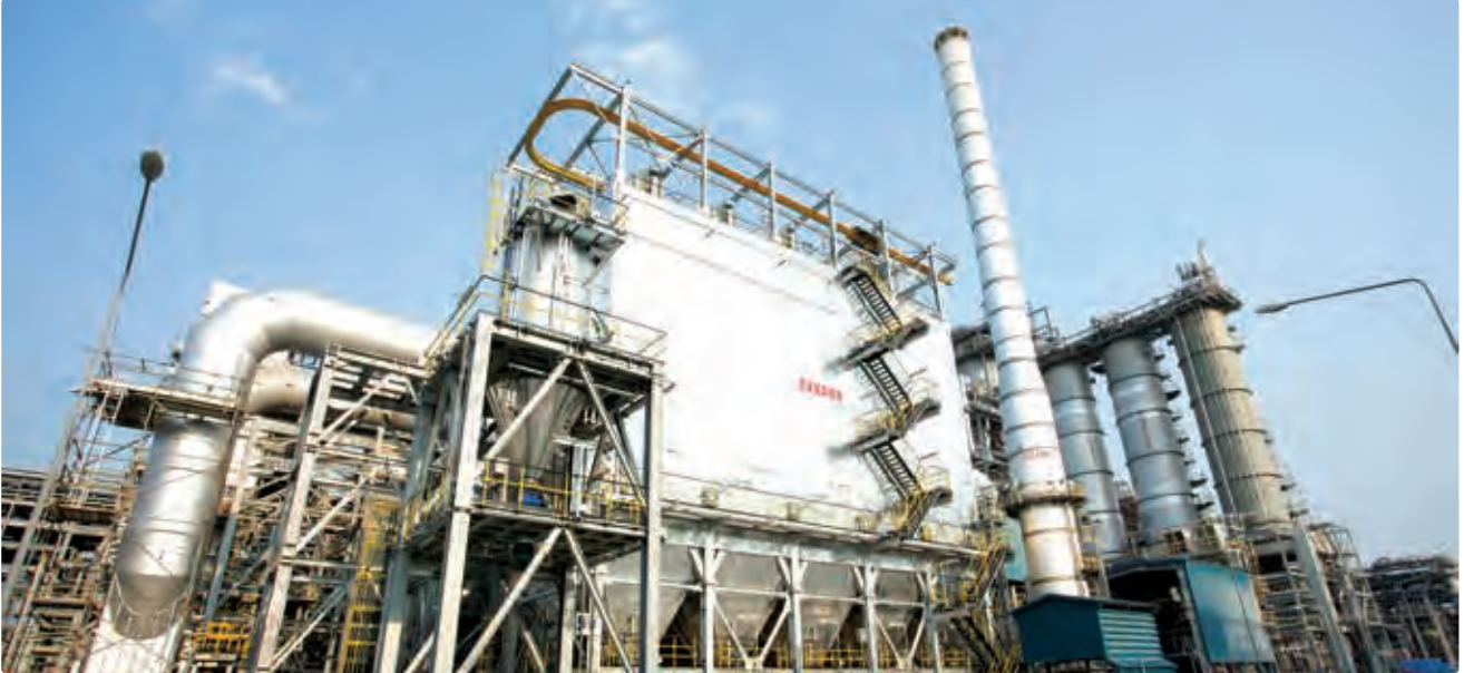
RDCC Unit 53 factory installed Electro Static Precipitator for higher efficiency micro dust collection.
